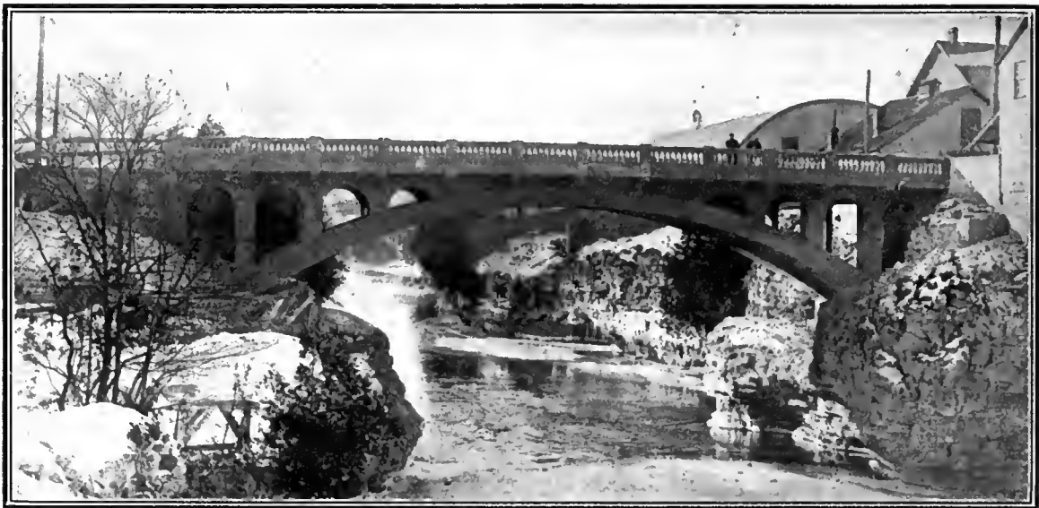
Tower Street Bridge, Fergus, Ont.
